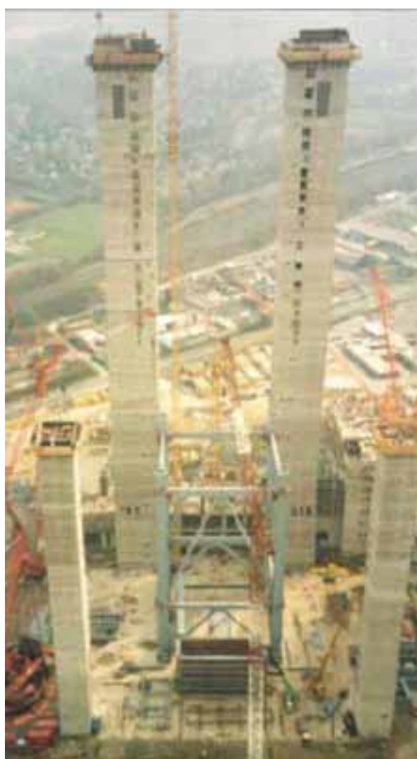
Aspect ratio d/b = 15.25\text{m} / 13.3\text{m} Slenderness h/b = 172\text{m} / 15.25\text{m} Total mass m \approx 24.100\text{t} Lowest flexural natural frequency n_1 \approx 0,30\text{ Hz} Critical wind velocity v_{crit,1} \approx 35,9\text{ m/s}
