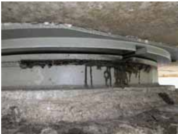
Fig. 3: (Chloride induced) corrosion damages of reinforcing or prestressing steel, leaky bearing element, bar tendon with missing grout
