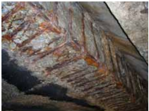
Fig. 3: (Chloride induced) corrosion damages of reinforcing or prestressing steel, leaky bearing element, bar tendon with missing grout
