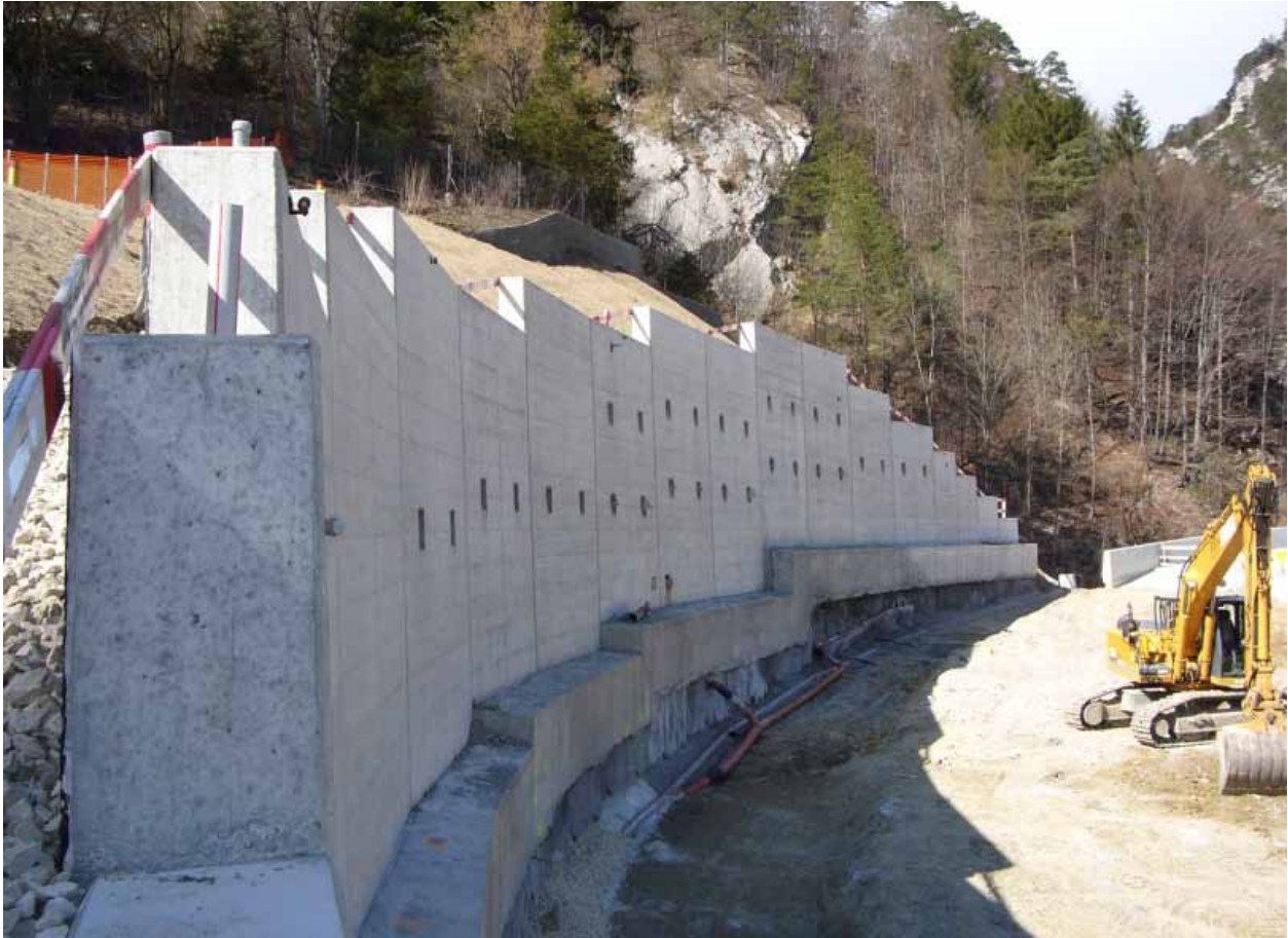
Figure 7: Court retaining wall, cross section and photo after completion
