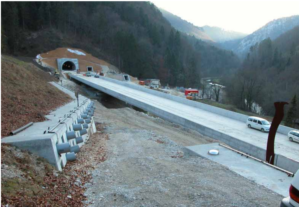
Figure 1: Parts of the Combe Chopin retaining wall
